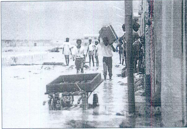
Streets in Male' were flooded during high seas which swept ashore in April 1987, washing away 30% of the capital island's reclaimed land.
